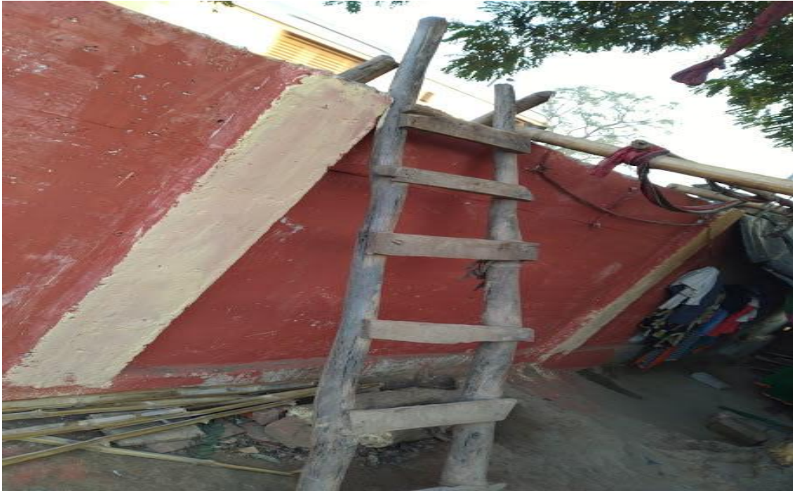
The wooden stairs at both the sides of a wall in Jalalpur Slum primarily is used for accessing the railway tracks to defecate
